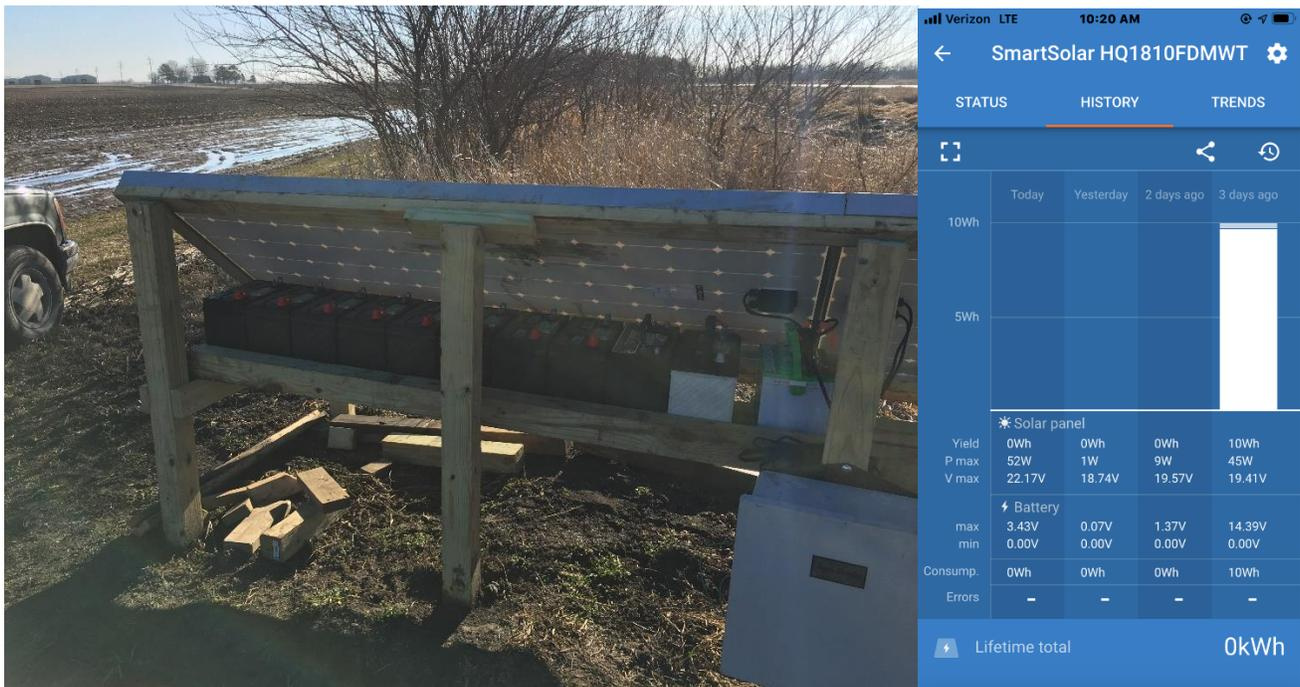
**Figure 1.** Solar panel and battery configuration for the Heat-Enhanced Bioreactor at the Agricultural Engineering Farm (Urbana, Illinois) (left) with the initial power and voltage read-out interface (right).
